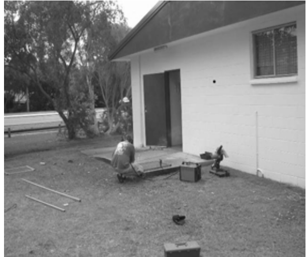
Peter (VK4TGV) fabricating security screens (2)
