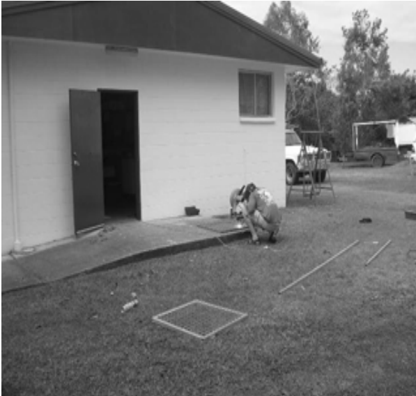
Peter (VK4TGV) fabricating security screens (1)
