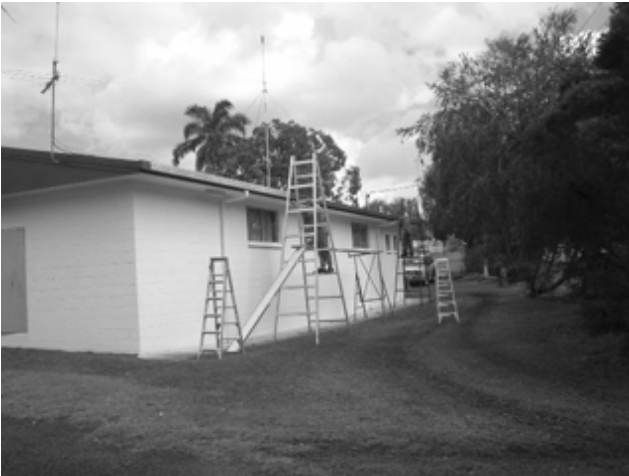
Finishing touches to the front guttering
